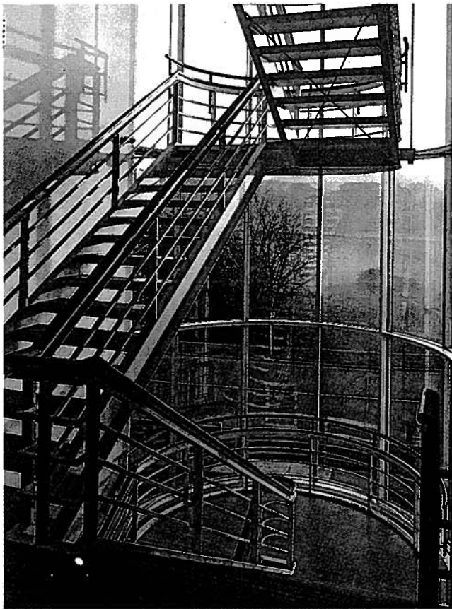
Left: inside the stair tower at the reception level on the second floor. Forcing the visitor to enter by stair or elevator "neither gives the visitor much of a lift, nor is it grand or inventive enough to be preamble."
